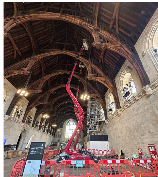
All electric MEWPs being used in Westminster Hall.
